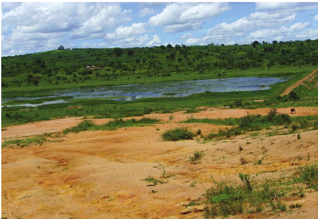
Plate 3: Soil erosion ridges around Kyambidde dam, Sembabule District
