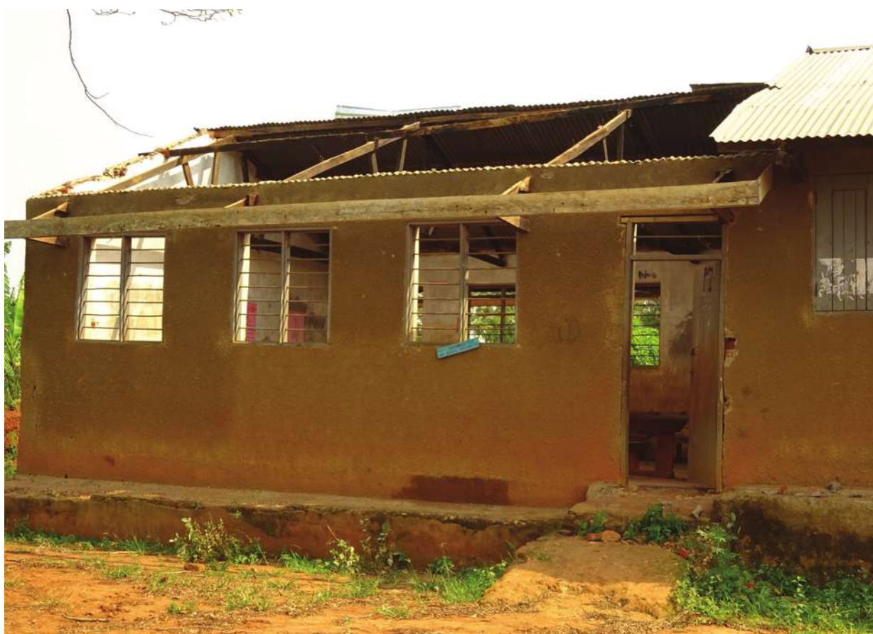
Plate 7: Strong winds impact, Njalwe Primary School in Lwemiyaga Sub county, Lubaale parish
